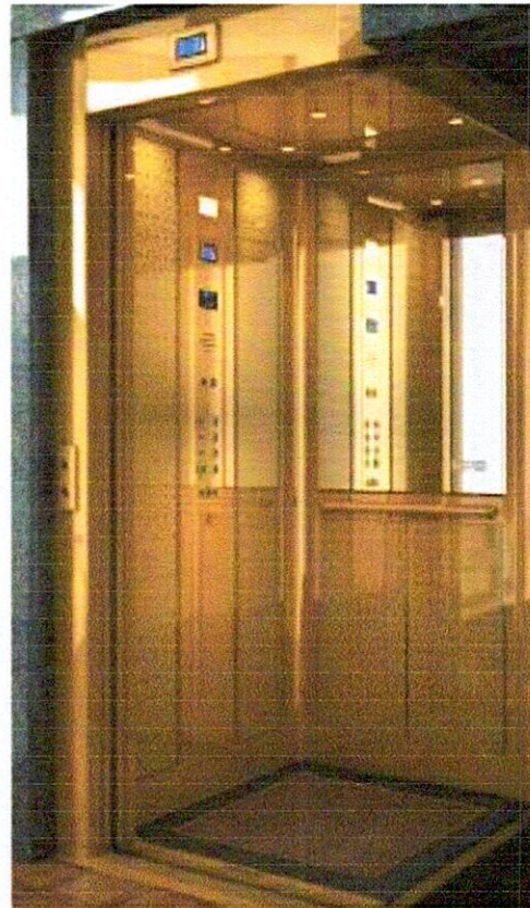
Accessible Elevator with Grab Bar, Mirror and auditory floor announcement system
