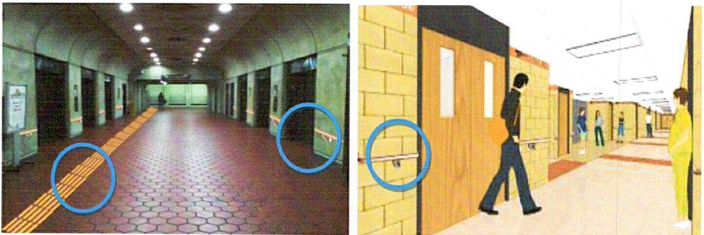
Accessible Corridors with Tactile flooring and low height grab bar as highlighted
