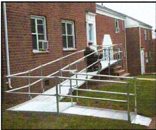
Accessible Ramp with Handrails for PwDs
