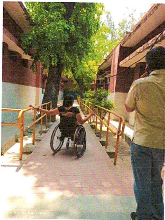
Main entrance for building with ramp and stairs (gradient 1:12)
