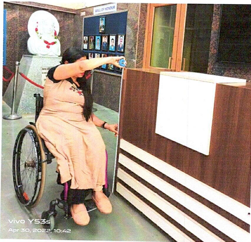
Inaccessible reception counter
