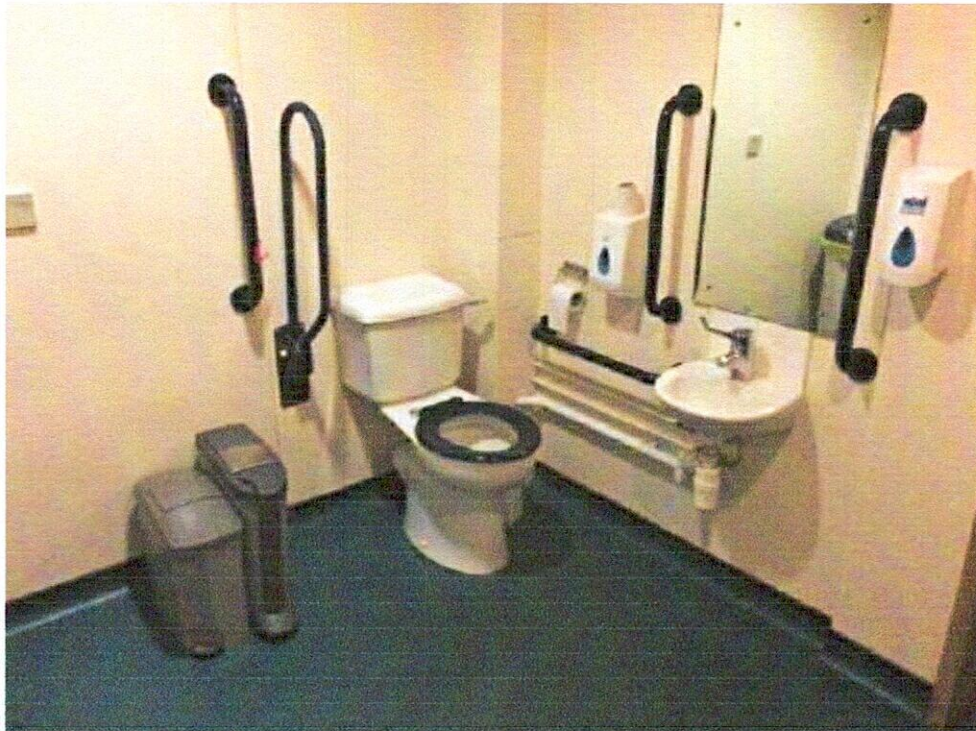
Accessible Toilets with Grab Bars
