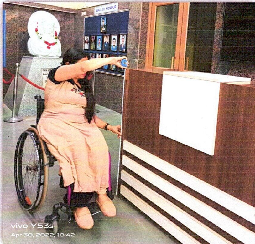
Inaccessible reception counter
