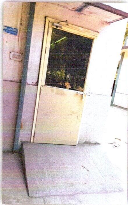
Ramps with railing and without railing
